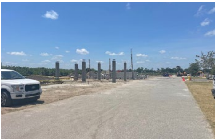
Slab done and walls going up at Concessions and Restroom Building.
